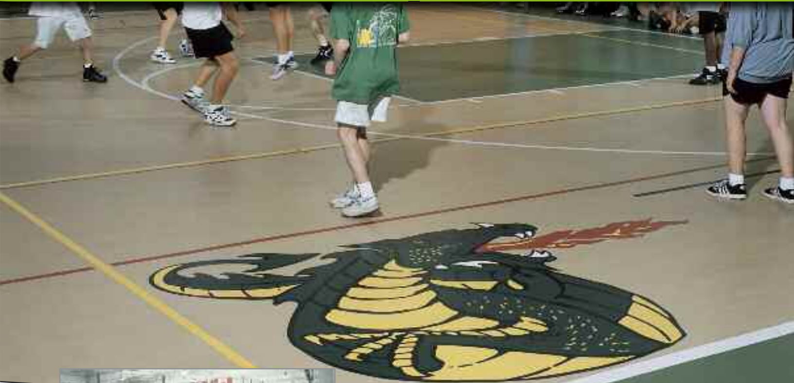
ElastoFloor™ poured urethane over pad – gymnasium floor.
