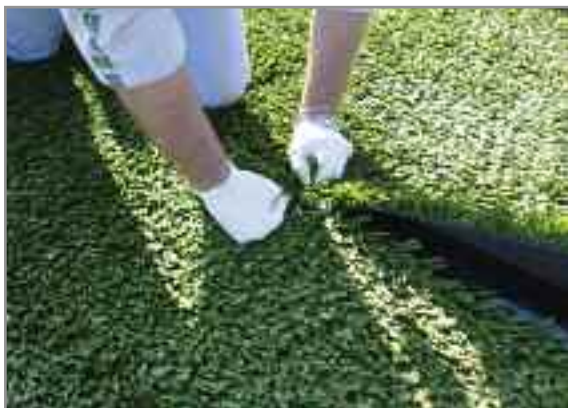
Ensuring tight seams.
