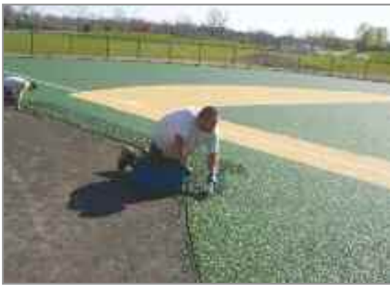
Applying the seamless rubber "turf."
