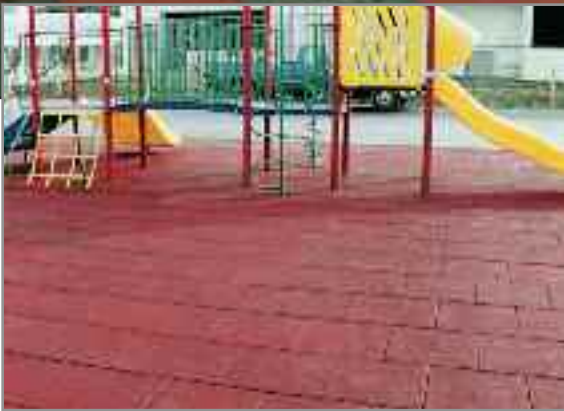
Staggered tile installation.
